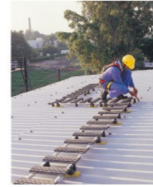
Roof Top Ladder
